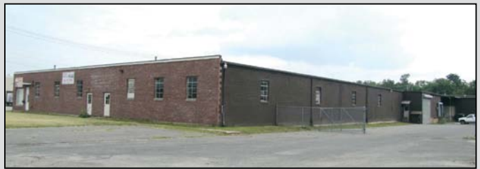
VIEW OF REAR OF BUILDING
