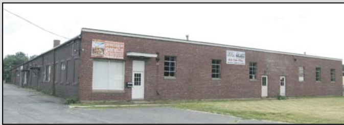
VIEW OF FRONT OF BUILDING
