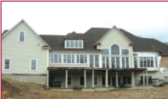
VIEW FROM BACK YARD
