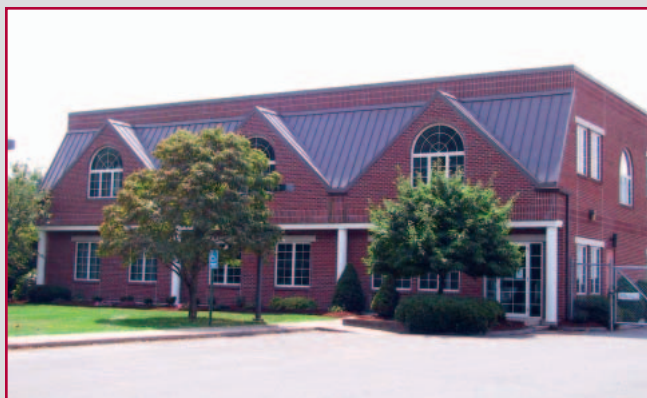
2 STORY OFFICE BUILDING
